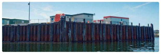
Photo 4. Completed Phase 1A Sheetpile Perimeter Wall around South Jetty
