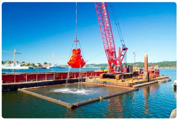
Photo 1. Phase 1B Dredging with Silt Curtain Frame
